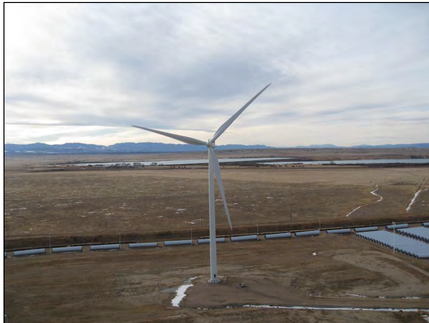
Figure B-3. Wind Turbine Under Measurement from Met Tower
