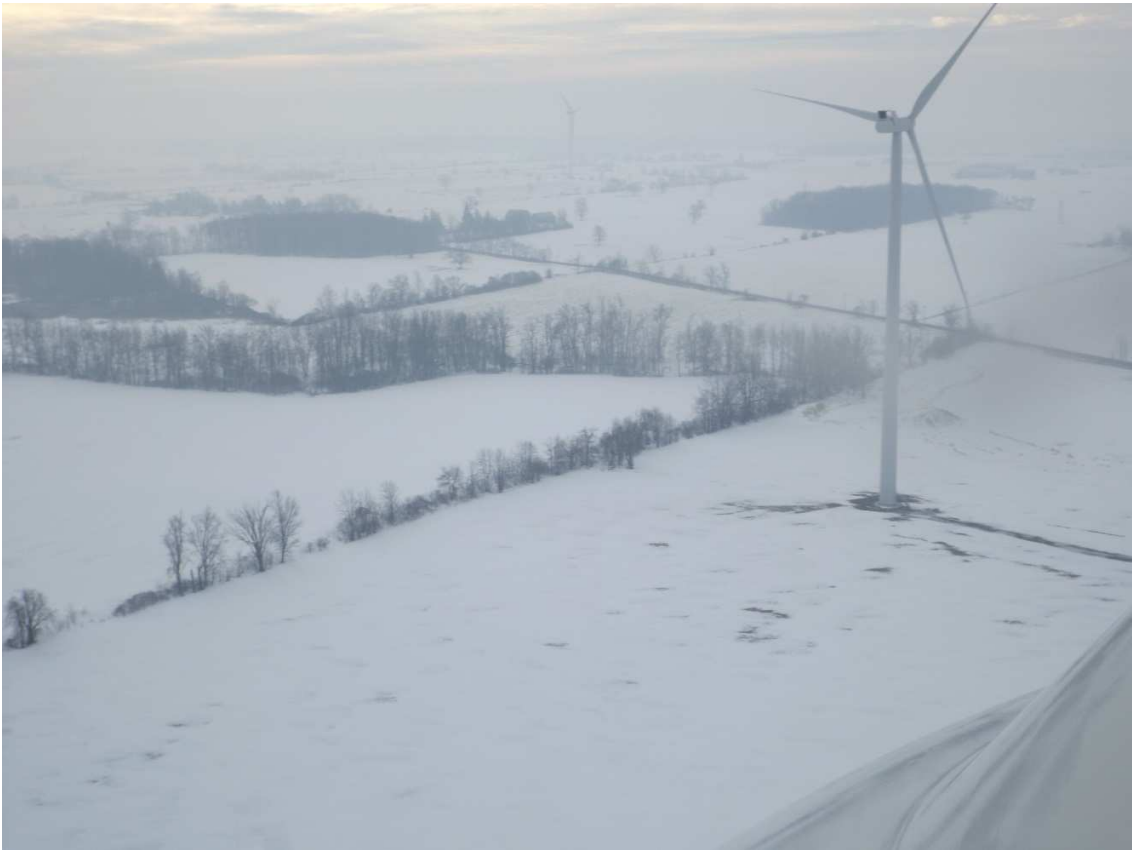
Figure 3. Overhead view of Turbine 2 Overlap. Picture taken from Turbine 1 Facing Southeast
