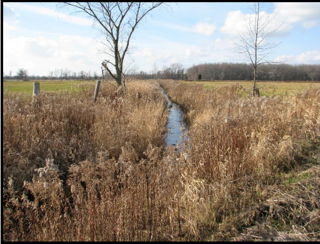
Casey Drain – south of Turbine 4 looking towards Station Road (winter)
