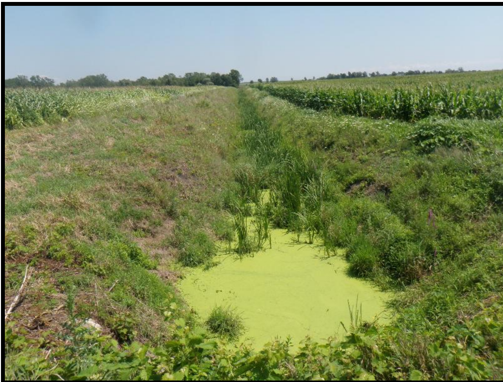
Crossing 4 – Feeder of Old Mill Race Creek looking east; south of Turbine 1 (summer)
